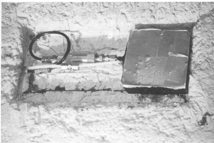
Figure 3 Photograph of piezometer embedded into anchor pile (courtesy of Walter Nold)
